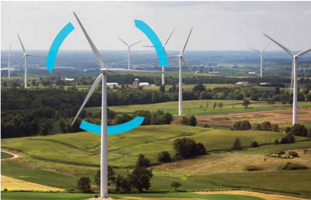
Viewing these windmills from the air, one can determine the wind is coming at us. The blades are turning counterclockwise.
